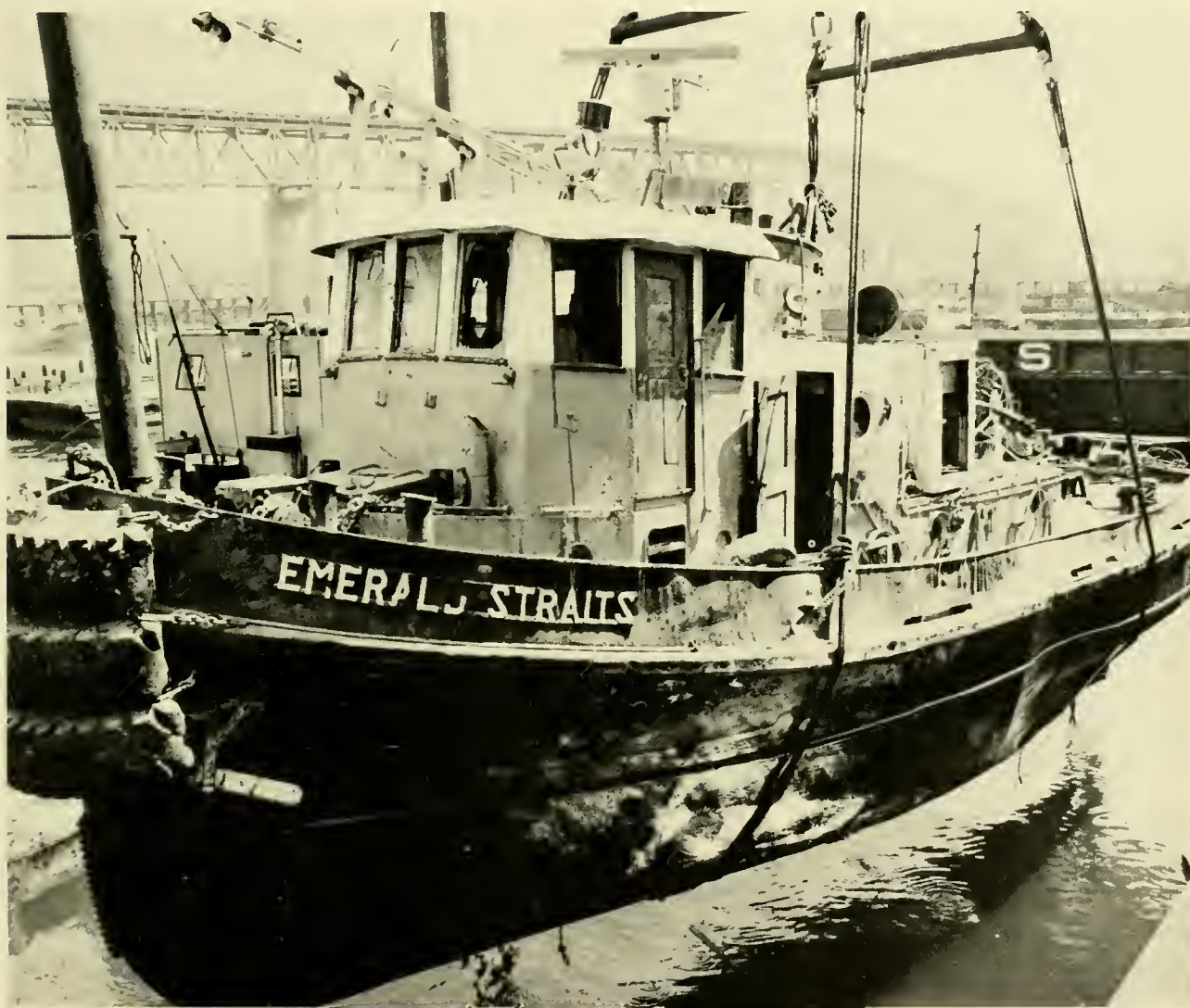
Fig. 11.24 The 95-ton EMERALD STRAITS . Retrieved from 670-foot depth in 1969 with lines attached by International Hydrodynamic's PISCES I . (HYCO)
