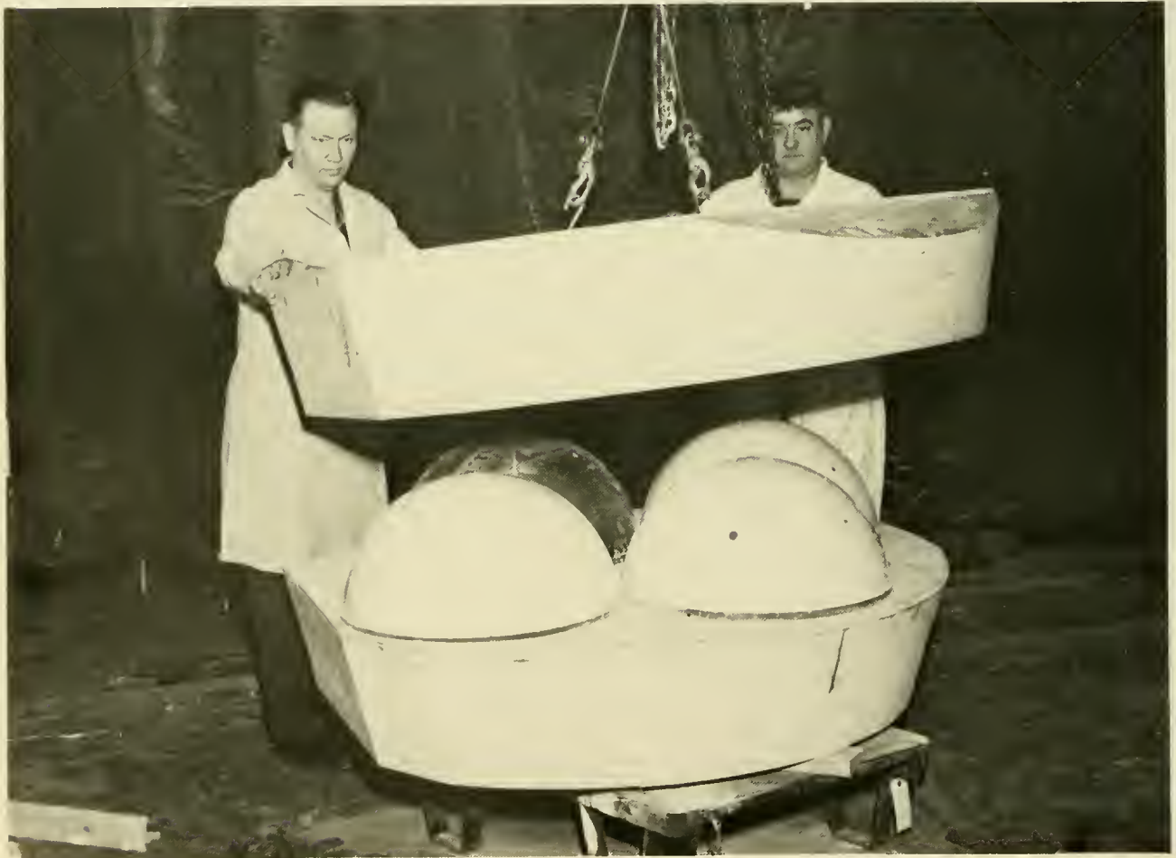
Fig 6.7 ALVIN's original buoyancy package consisted of syntactic foam and aluminum spheres. The total package provided 4,000-lb positive buoyancy (WHOI)
